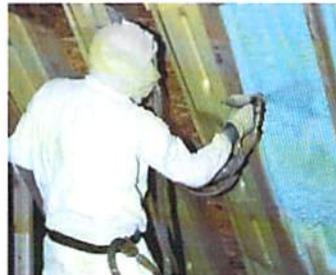
STYROFOAM™ SPF Insulation meets IBC/IRC requirements for foam plastic insulation and is UL Classified Class I at 4 inches (UL 723). Also see ASTM C1029 and ASTM E84.
